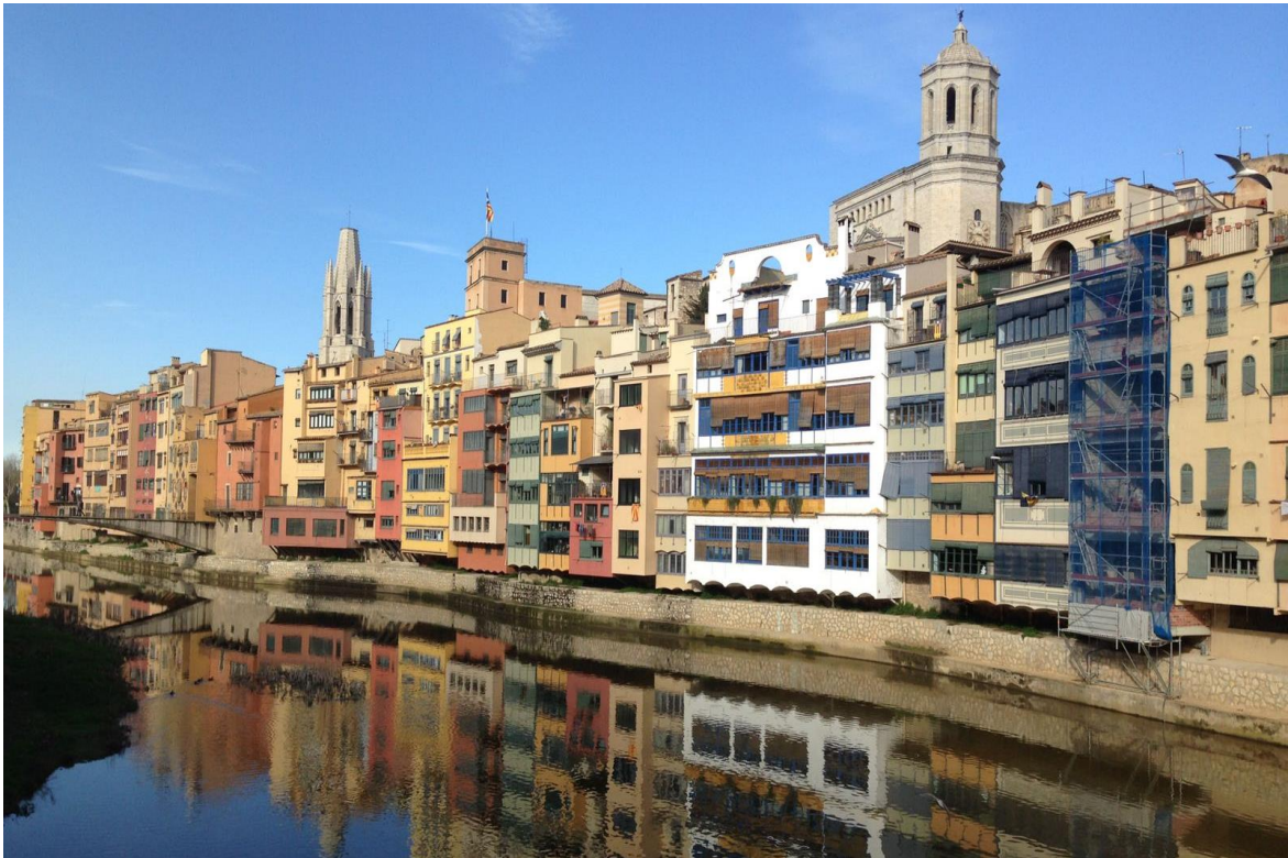
Figure 4 The coloured house on Onyar river (Credits to Mark Urkiza)
