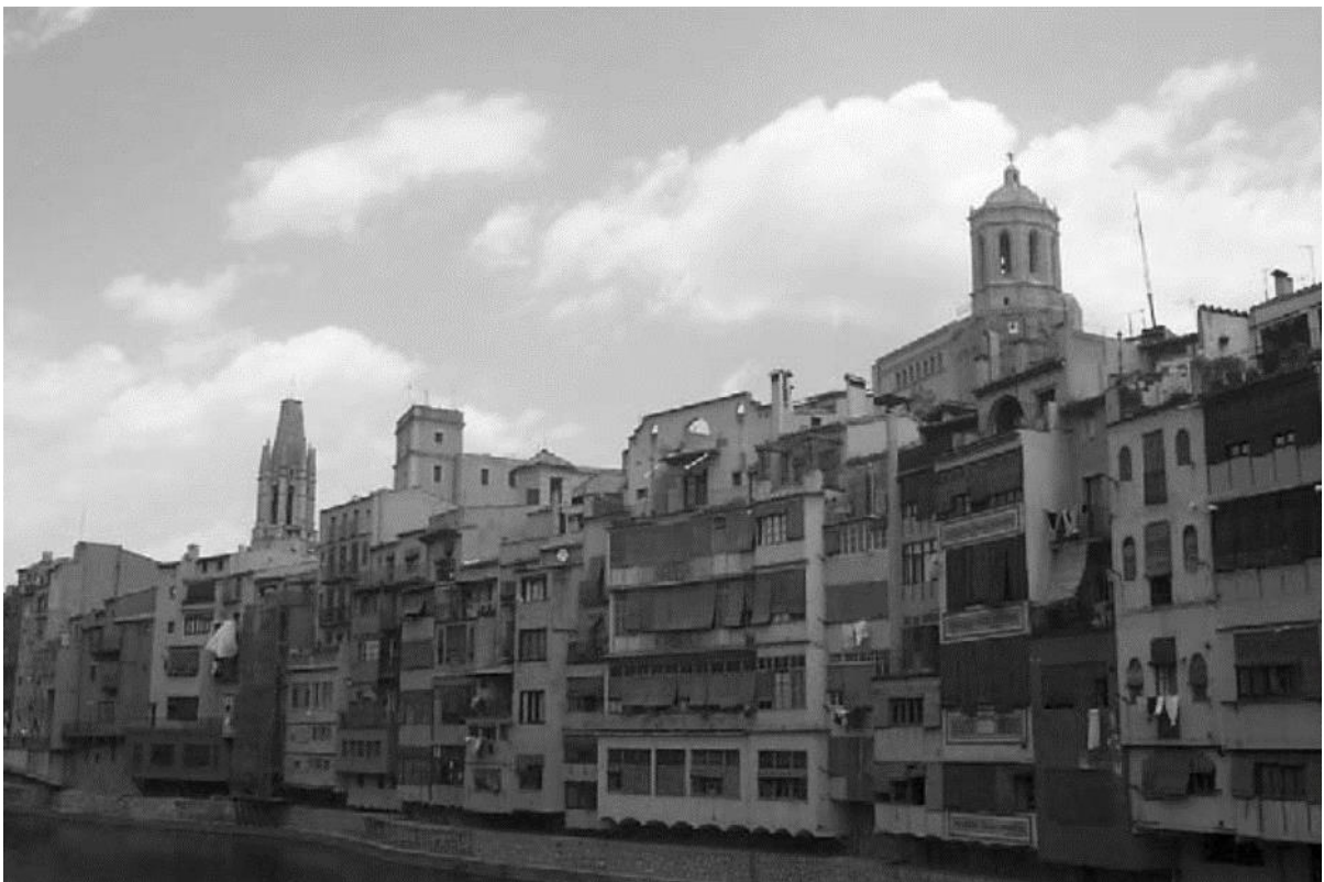
Figure 1 the houses on the river Onyar River (Taken from Galì and Donaire, 2005)
