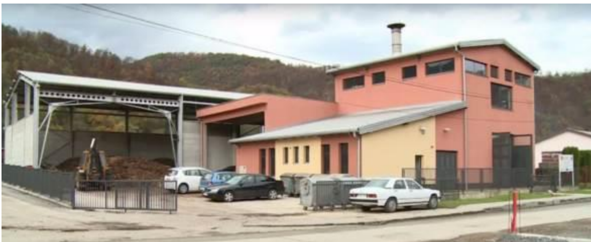
Figure 6. The existing biomass heating plant in Nemila
