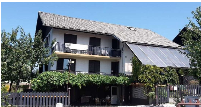
Figure 17. South-Facing Side of the Case Study Building
